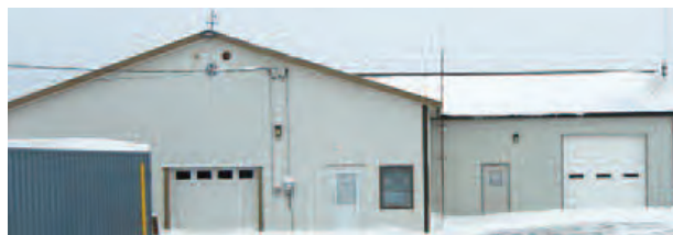
Our staging building, used to house exhibit creation and repair facilities, now also serves as temporary artifact storage. The green container at left holds more temporary storage.
